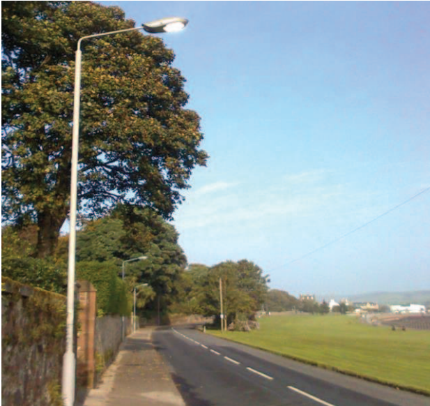
Replacement LED street lighting installed in Kilkerran Road Campbeltown. Works consisted of installing new columns, LED lanterns and new ducting and cabling.
