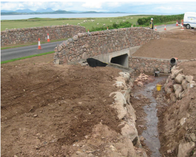
New Bridge constructed on A83 just north of Muasdale in Kintyre in July/August 2013
